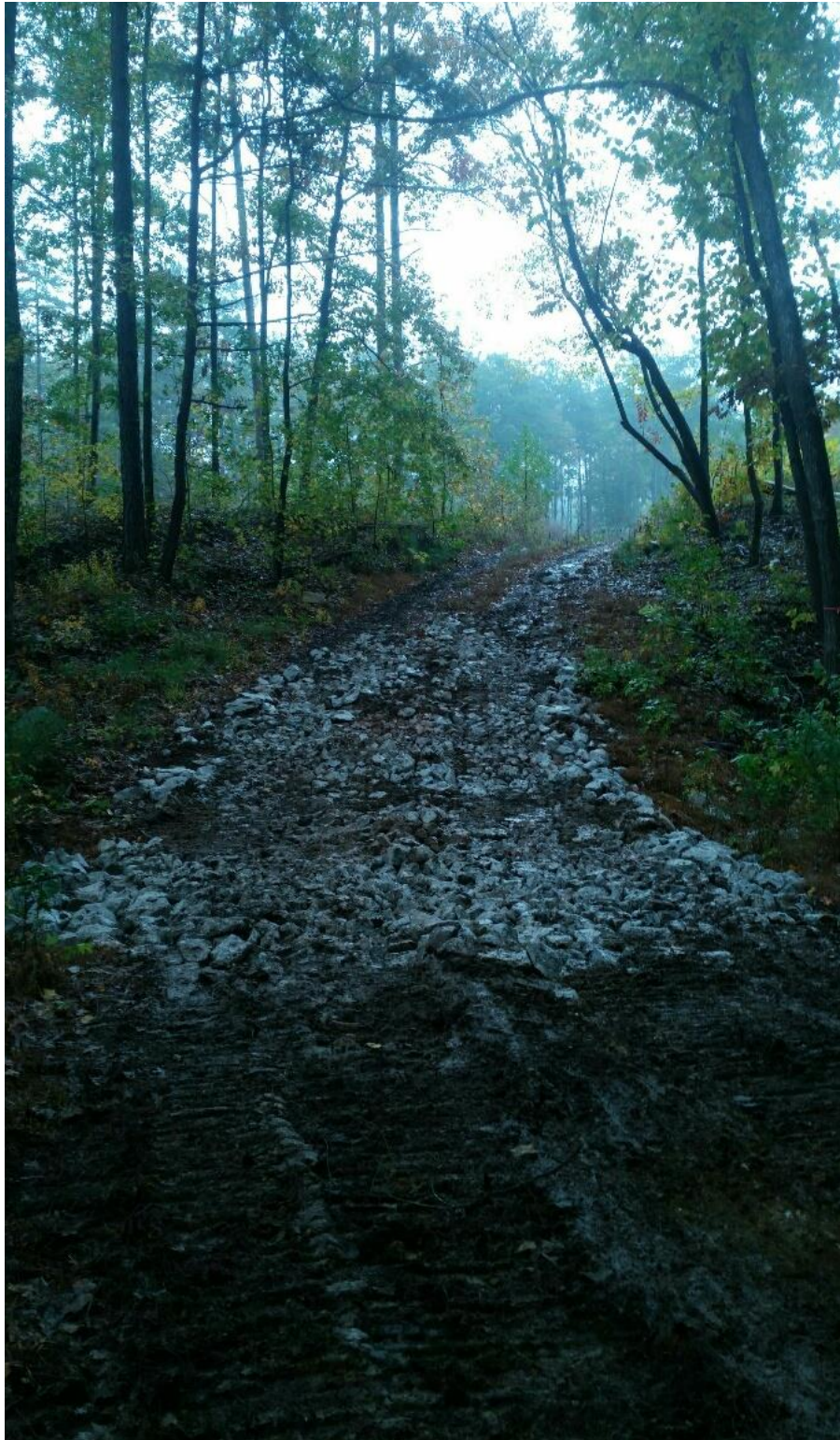
T24A - Reinforcing Steep Slope at Area 11 to Alternate LWC
