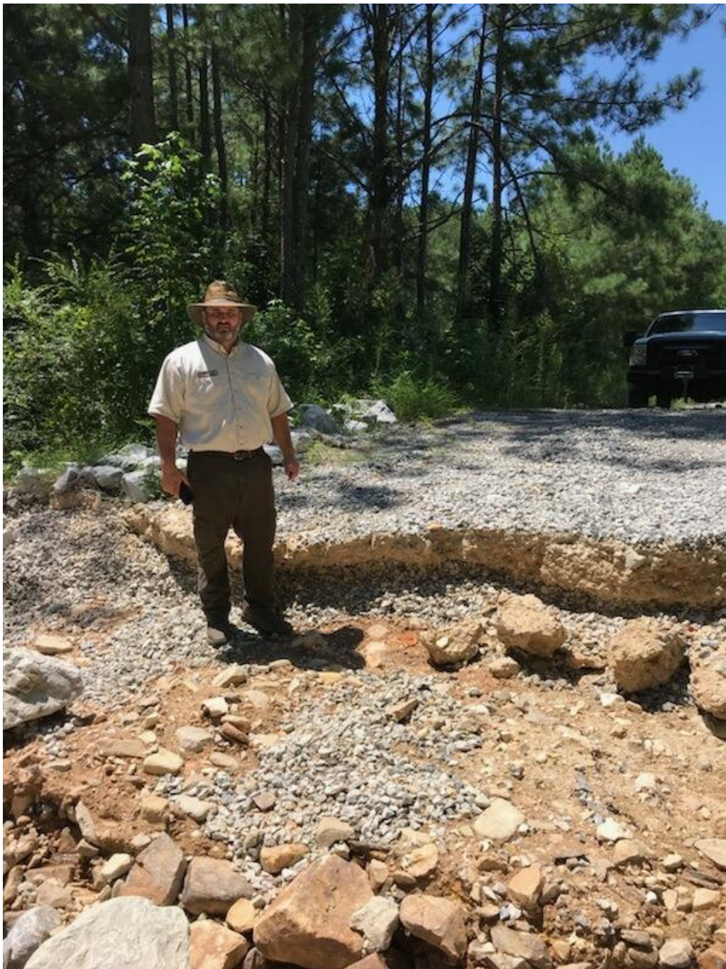
T24A - Washout of Original Low Water Crossing
