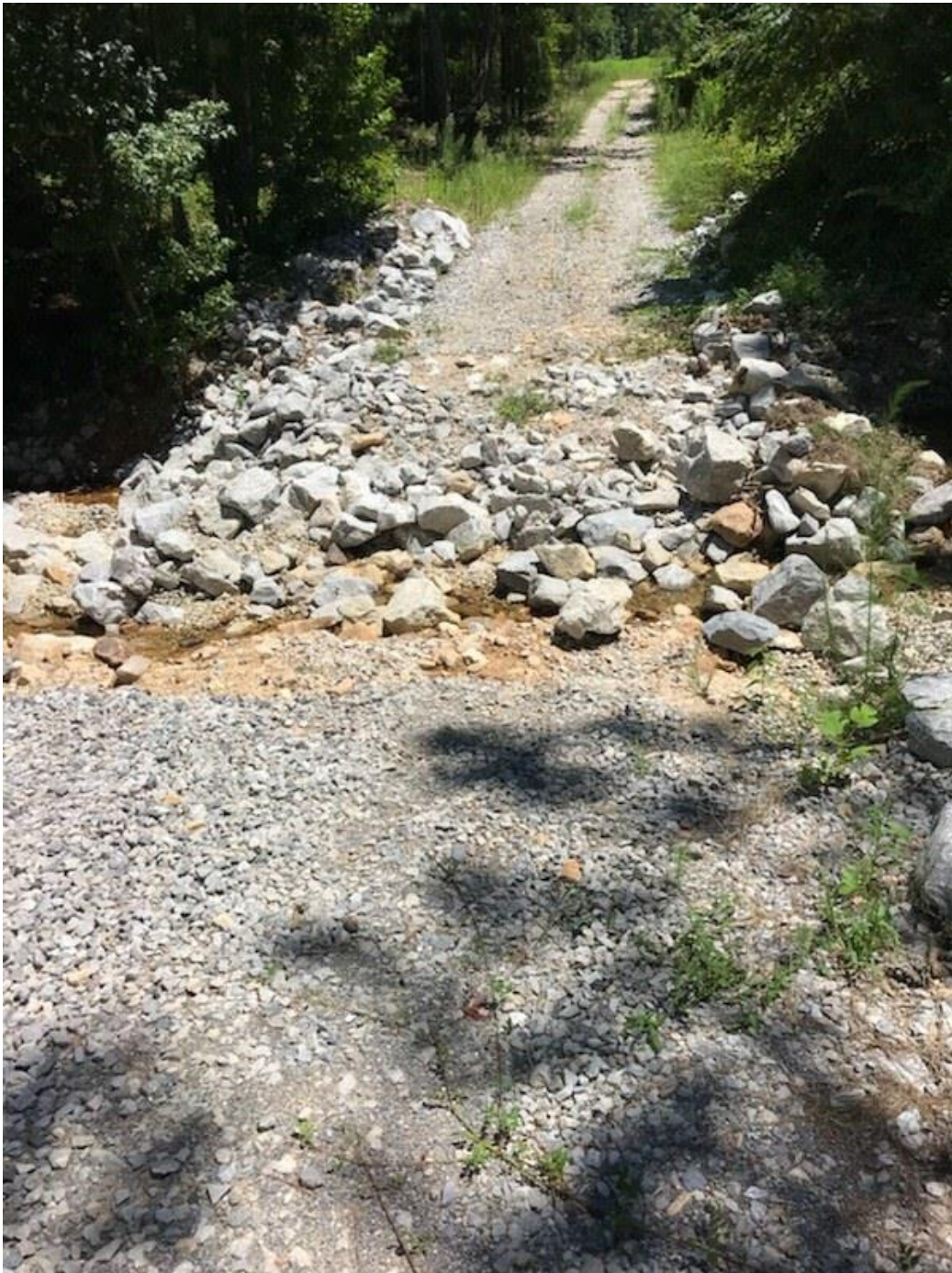
T24A - Washout of Original Low Water Crossing
