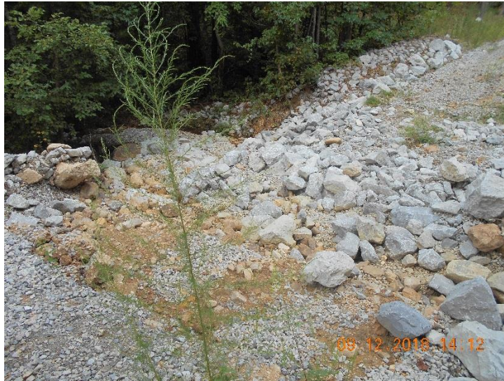
T24A - Washout of Original Low Water Crossing
