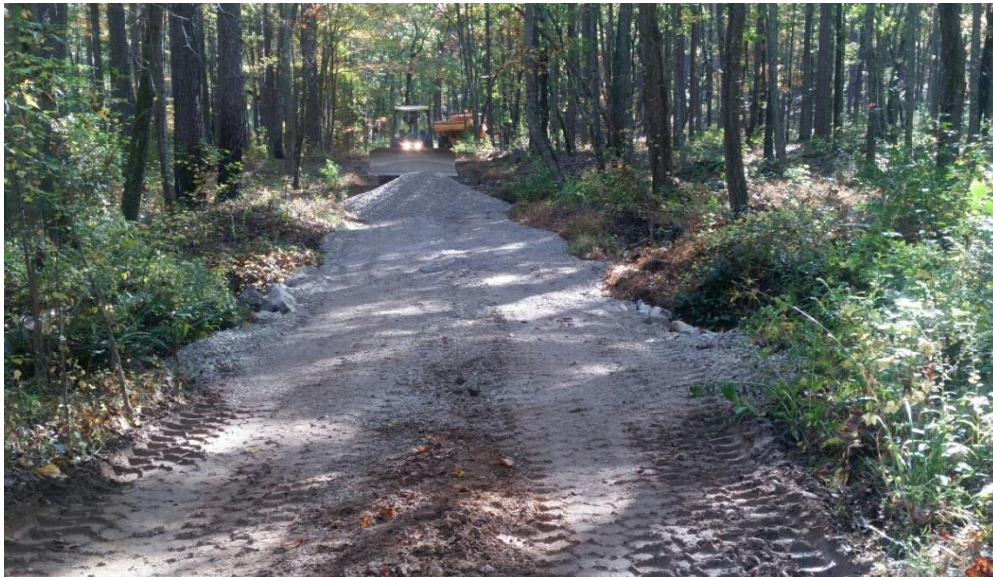
T24A – Clearing and Reinforcing Back Road to Alternate LWC
