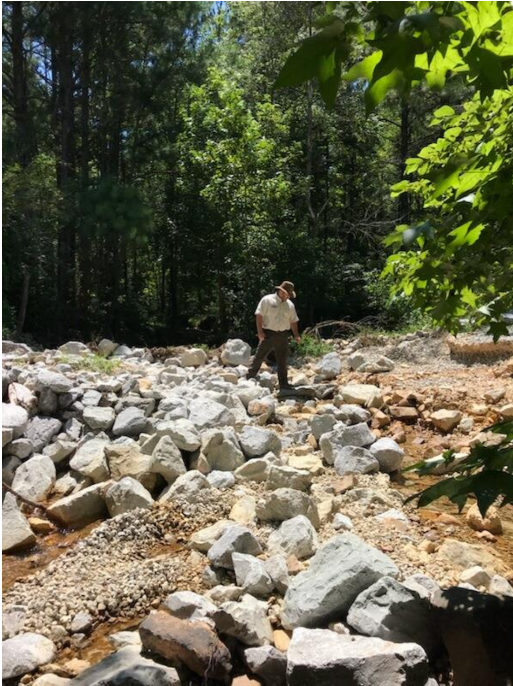
T24A - Washout of Original Low Water Crossing
