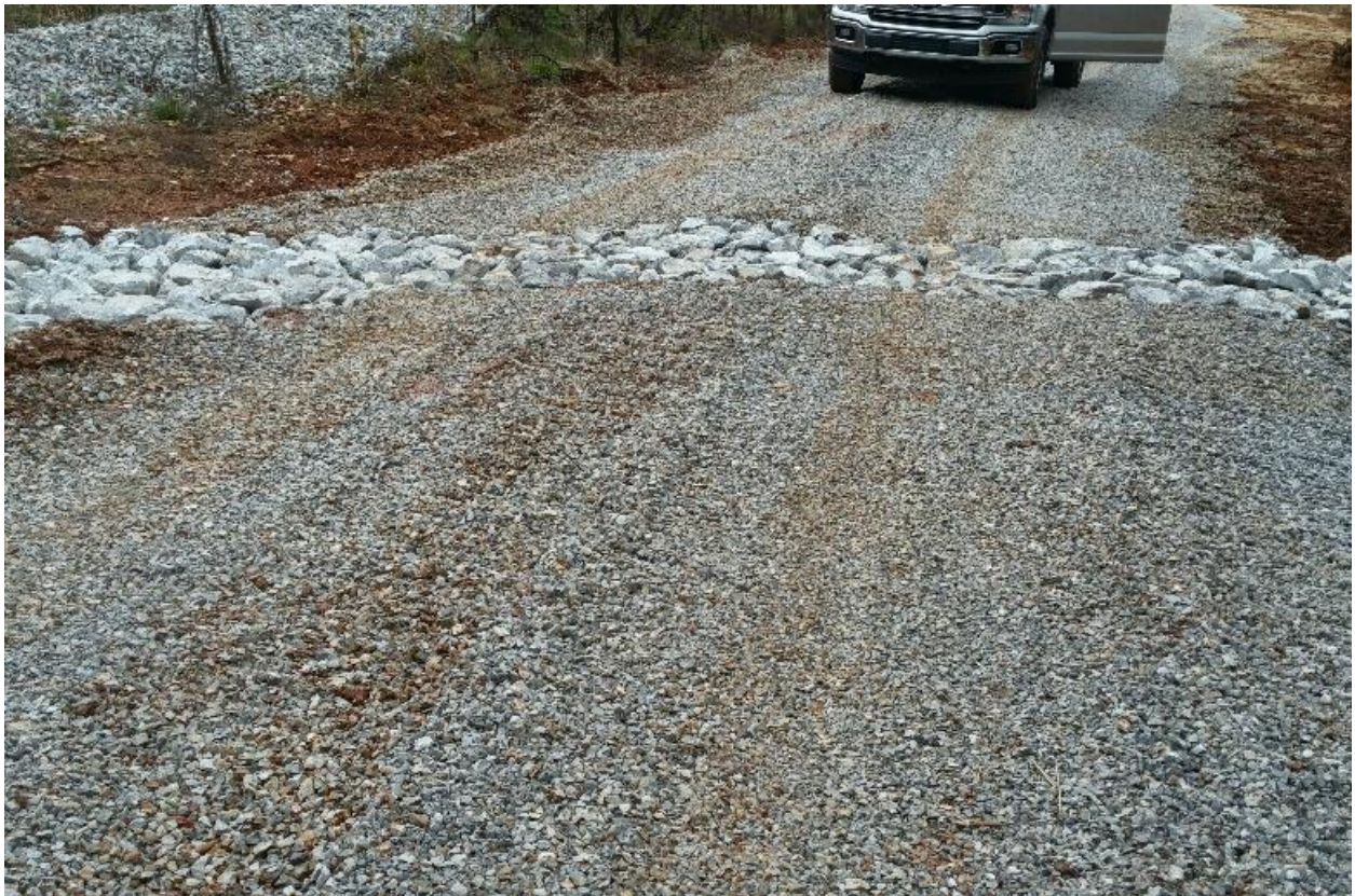
CCR – Repair of Haul Road Near Area 4 with Riprap Drain
