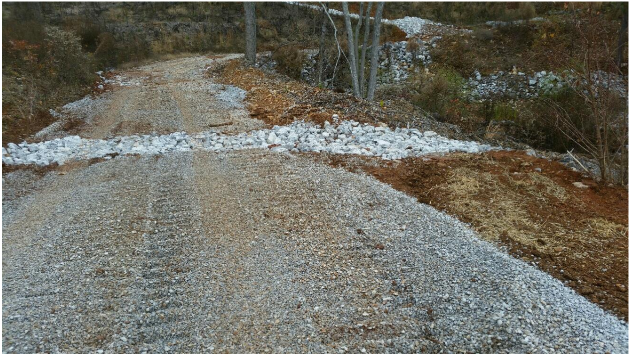
CCR – Repair of Haul Road Near Areas 1/3 and 2
